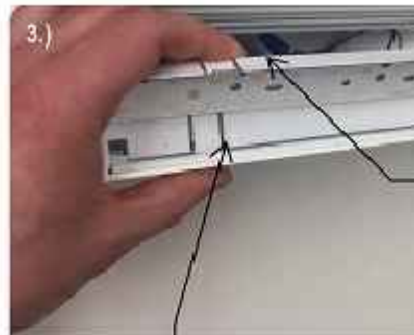
3.) LOCATE GROOVE TO REINSTALL REFLECTOR
